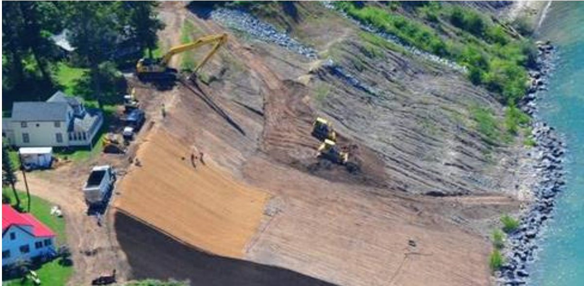
Figure 6.6B: Mitigation methods being adopted at this site include toe protection using riprap, slope re-grading to a dual-slope configuration, installation of koir matting and erosion-control matting, vegetative plantings, septic-system modifications, and ground- and surface-water interception drainage (Images: modified from www.lakebluff-ny.org ).
