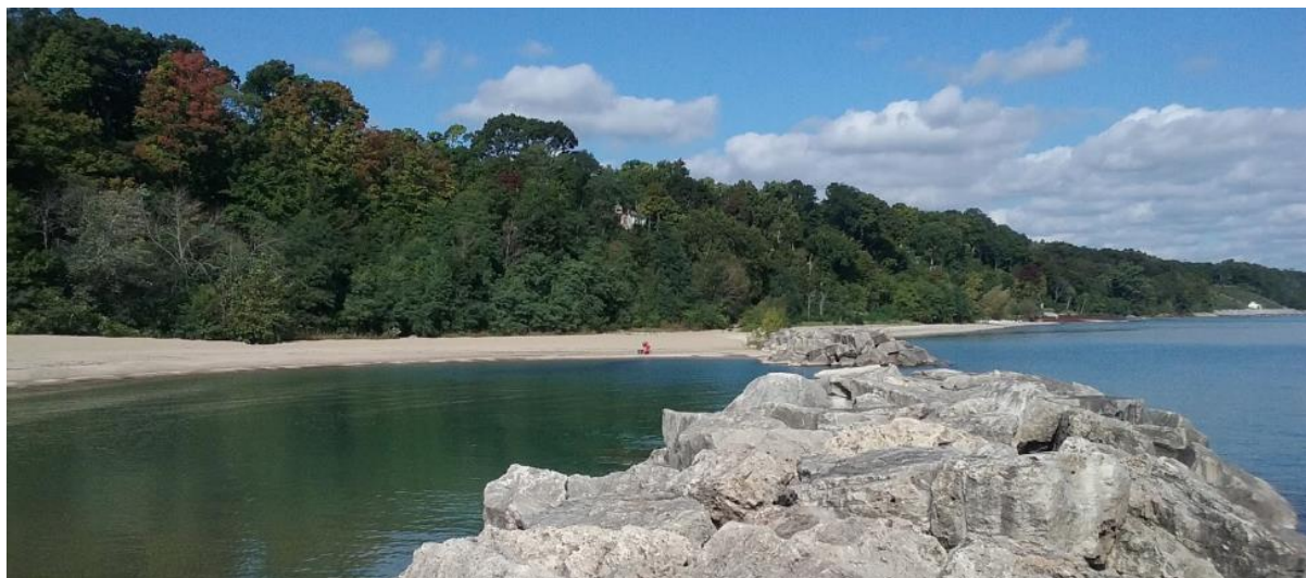
Figure 6.10: Forest Park, Lake Forest, Illinois, near Chicago. This is an example of an attached offshore breakwater design on the Lake Michigan bluff coast that provides beach resources, a safe harbor, and bluff stabilization. Littoral drift moves from north to south. Note erosion mitigation using bluff slope reduction in the far distance in the lower image (Images: maps.google.com).
