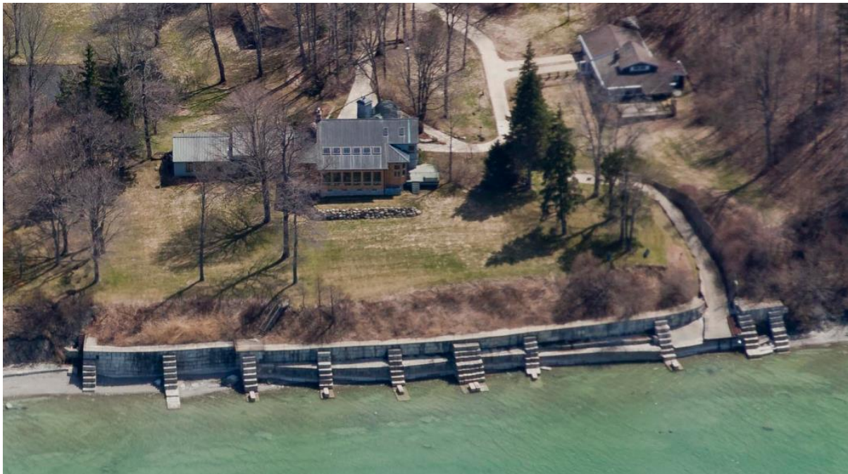
Figure 6.25: Buttressed, dual-level, curvilinear (in plan view) concrete-cube bulkhead resting on beach or bedrock in western Erie County. Stepped buttresses allow lake access from the bulkhead and function as short groynes to allow seasonal beach accumulation (April 2015 imagery, available from PA DEP Coastal Resources Management Program at http://www.dep.pa.gov ).
