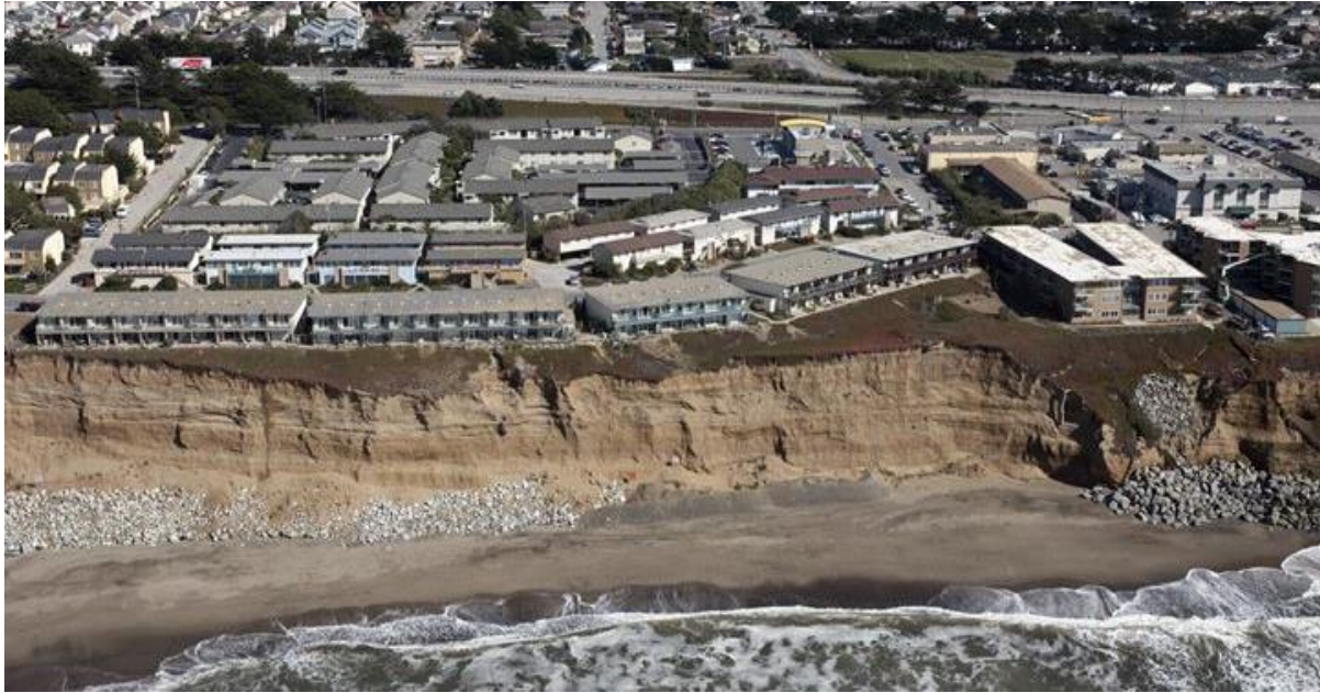
Figure 6.8A: Oblique aerial photograph (from 2009) of the pre-1970s Esplanade Apartments complex, Pacifica, California. The image illustrates chronic bluff failure (debris falls, gullying) in an urbanized setting where five apartment complexes sit atop sandy Pacific coast bluffs. Sufficient time may not have been available at this site to develop a proactive erosion-mitigation plan. Hard stabilization (riprap) placed at the bluff toe is not preventing continuous bluff retreat at the site.
