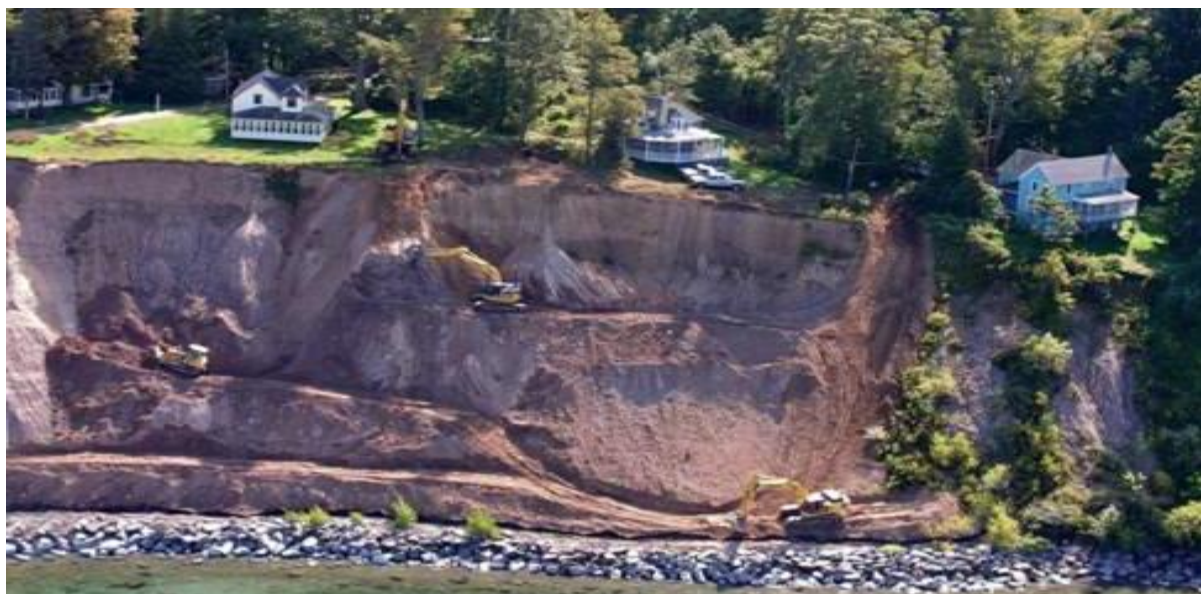
Figure 6.6A: Example of proactive mitigation of a bluff-retreat problem on the Lake Ontario coast at Lake Bluff, Town of Huron, New York, using a comprehensive approach to address several causes of historical bluff instability. The stratigraphy at this New York site is similar to that of the Pennsylvania coast.
