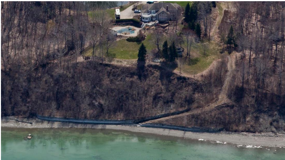
Figure 6.17: Stacked concrete-cube bulkhead west of Sixteenmile Creek, eastern Erie County. The bulkhead rests on beach or on shallow bedrock beneath the beach (April 2015 imagery, available from PA DEP Coastal Resources Management Program at http://www.dep.pa.gov ).
