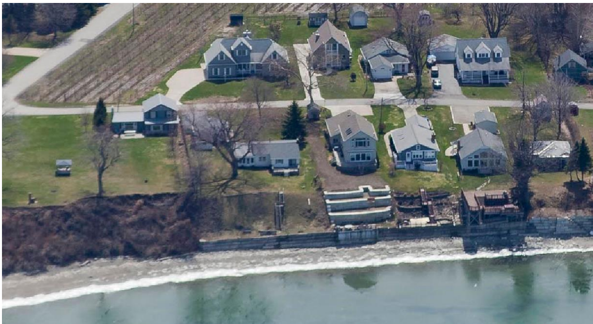
Figure 6.15: A bluff-toe bulkhead and terracing, using concrete cubes, protect a low bluff in eastern Erie County. A bedrock toe is absent at this location (April 2015 imagery, available from PA DEP Coastal Resources Management Program at http://www.dep.pa.gov ).
