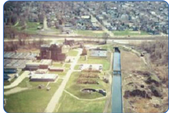
Erie's Wastewater treatment plant and the Millcreek Tube
