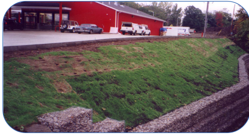
Streambank stabilization
