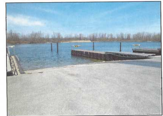
Presque Isle State Park. Boat Launch improvements at the Marina included the lengthening of concrete pads and shoreline stabilization. DEP file photo.
