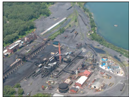
Figure 14. Coking plant located on the Lake Erie shoreline
