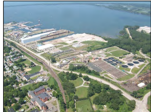
Figure 4. Erie Wastewater Treatment Plant
