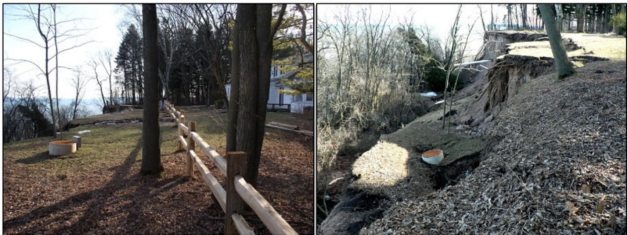
Figure 2.7. Septic system lost during a bluff retreat event along the Lake Michigan coast. Image on left was taken January 1, 2006 and image on right was taken March 20, 2006 following the slumping event (Credit: Barry Sullivan, Ozaukee County; https://greatlakesresilience.org/case-studies/land-use-zoning/minimizing-bluff-top-development-risk ).
